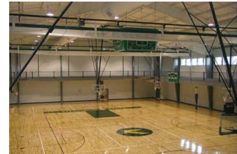
Athletic & Recreational Facility at Fitchburg State College Fitchburg, Massachusetts
