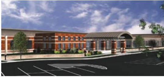
Renovations to Building 1614 at Hanscom Air Force Base Bedford, Massachusetts
